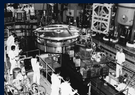
Institute Laue Langvin, remote 6 axis underwater reactor cutting machine
